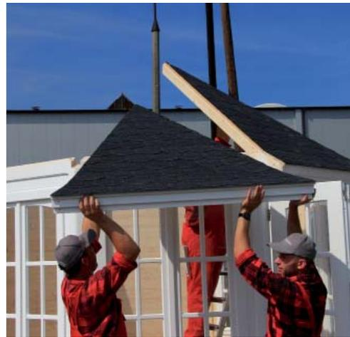
The provided roof elements are generally inserted into the already assembled wall. Set all roof elements (the roof elements show here come pre-shingled) carefully on the provided tongue of the exterior walls. Support the pieces in the centre of the pavilion. Use a ladder; this will also help you when you lay the roof elements on the walls. After laying all roof elements, they will support themselves so that the roof cannot collapse.
