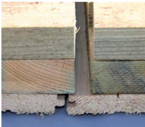
Set the two preassembled floor elements upside down on the foundation. Push the two floor elements together so that groove and tongue are closed in the centre. Make sure both pieces are flush on the sides.
