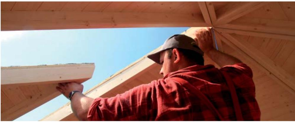
Now take a screw clamp and tighten the adjusted roof element at the roof overhang (outside) and screw them together from the left and right hand-side. Place two small pieces of wood underneath the clamp to protect the wood.
