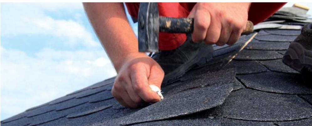
Start at the bottom of the eave and lay the first shingle centred on the ridge (roof edge) so that half of the shingle covers each side. Nail the shingle to the roof using two roofing nails in the upper half of the shingle. Place the
