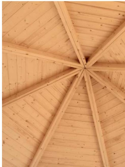
If necessary, adjust the position of the roof element with a hammer. After screwing all roof areas on the outside, the elements need to be aligned at the top. Do this by pressing or gently hammering from the outside (one person on the roof). Screw all elements together one by one.
