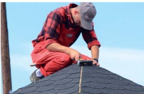
Make sure the adjoining roof beams are flush when adjusting the pieces. Screw all roof elements together properly and to the wall elements.
