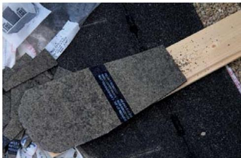
In our example the individual roof areas are already shingled, which means you only need to attach some small pieces of roof felt to the roof edges (ridge).
