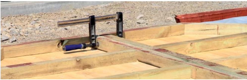
Now take screw clamps and fix the floor elements where they meet and screw them together with the provided screws (approx. 6-8 screws depending on the model).
