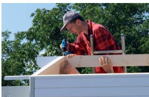
Now screw the fascia rails and the ridge purlin to the respective components with the proper tension.
