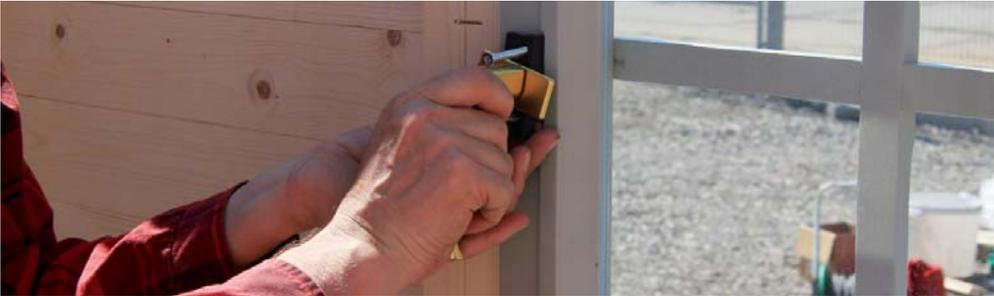
You can screw in the bottom screw after opening the window since the window handle will not get in the way anymore.
