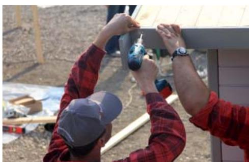
The roof boarding is already cut to the correct length so that you only have to lay the boards from front to back.
