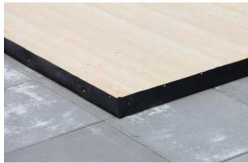
If you also want to protect the floor with roofing felt, pull up the excess material and fix it to the fascia boards of the floor with small nails or staples. Cut off any remaining excess material with a cutter.
