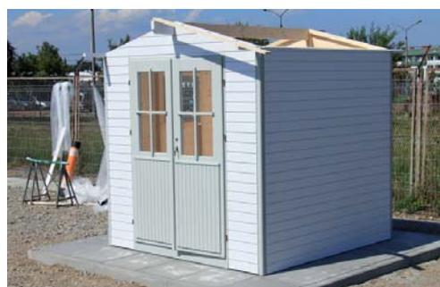
Make sure that the spacing of all inserted boards is the same. In the next step, you will mount the roof boarding.
