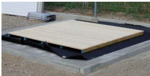
Set the preassembled floor in the desired position on the foundation.
