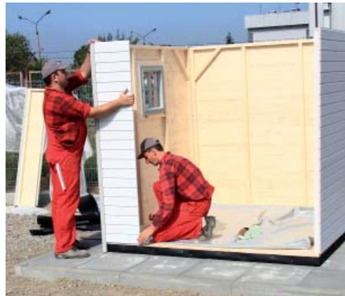
Now place all wall components, one after the other, where they belong as shown in the drawing. Screw the wall components at least 4 times per side (on top, at the bottom and twice in the middle with the appropriate spacing).
