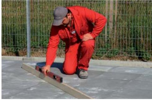
As a basic principle, only build your summer house on a level surface. Check your foundation prior to assembly!
