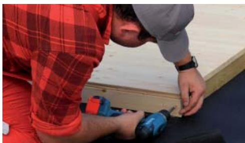
Fix the two missing fascia boards of the floor with a cordless screwdriver and the provided screw set.
