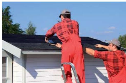
Lay the sheets so that the next layers always overlap the underlying sheet at the upper edge by approx. 20-30 cm.
