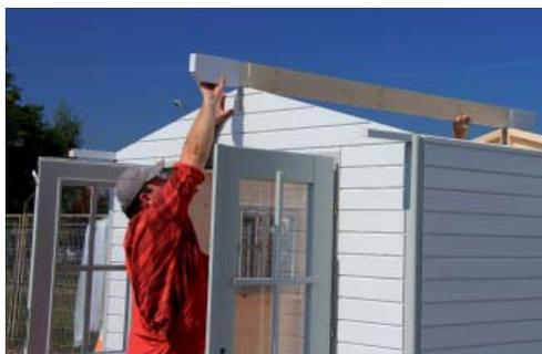
Now place the ridge purlin in the prefabricated slots. Attach the two fascia rails on the left and right hand-side of the gable.
