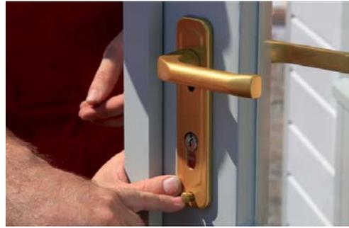
Insert the window handle into the lock in the window. Use a cordless screwdriver or a screwdriver to screw in the uppermost screw.
