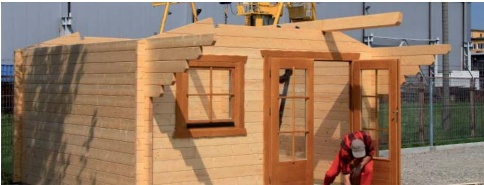
The ridge planks for the front and rear part of the summer house are already preassembled. Take the first two pieces and set them on the exterior walls in the front and back. Make sure the planks are attached properly. If necessary, tap the left and right-hand side of the gable with a hammer to make sure it is attached properly to the wall. This also applies for the rear gable.
