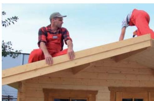
Mount the **fascia boards** with screws to the roof boarding.
