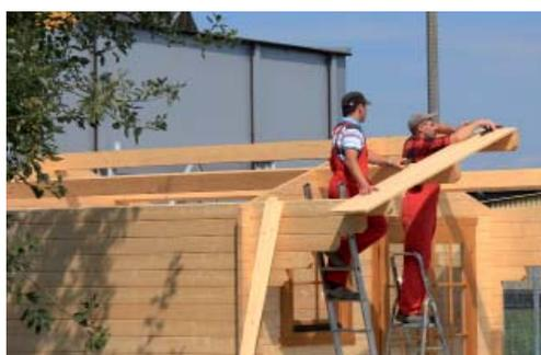
Now nail the boards twice to the ridge/centre purlin and the fascia board. Lay the roof boarding all the way to the back. Measure in regular intervals to ensure that they are properly aligned and that the spacing to the wall is consistent. The backmost (final) board needs to be cut to size in most cases.
