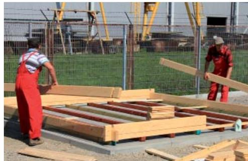
Take a plank for the front and back, and then a plank for the left and right-hand side, continuing to alternate in this fashion. Carefully assemble the pieces, ensuring they are properly interlocked using the provided block of wood. Always check the number of assembled plank rows against the number in the drawing to prevent errors.
