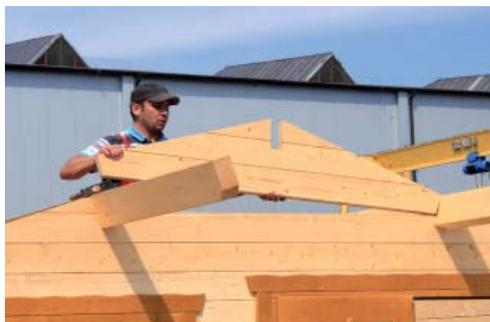
Insert the two centre purlins into the slots in the gable. Make sure the beams (purlins) are flush and at the same angle with the gable. Adjust them with a hammer if necessary. Now set the second (smaller) piece of the gable between the two centre purlins and on the already assembled front part of the gable. Repeat this step for the rear gable. Then insert the ridge purlin into the upper slots of the gable.
